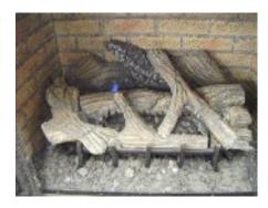
The pilot is located in the back left of the unit.
