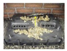
The pilot is located in the back of the unit.
