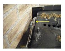
Pilot assembly is located on the left side.
